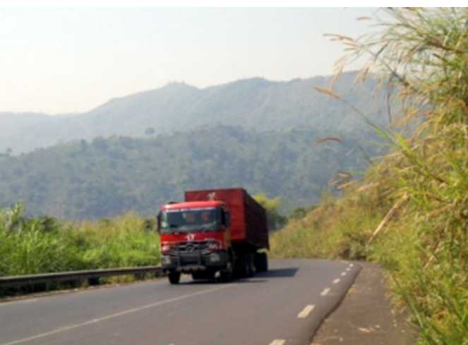
Photo 3 - Environmental maintenance is needed on Cameroon's Mélong-Dschang road
